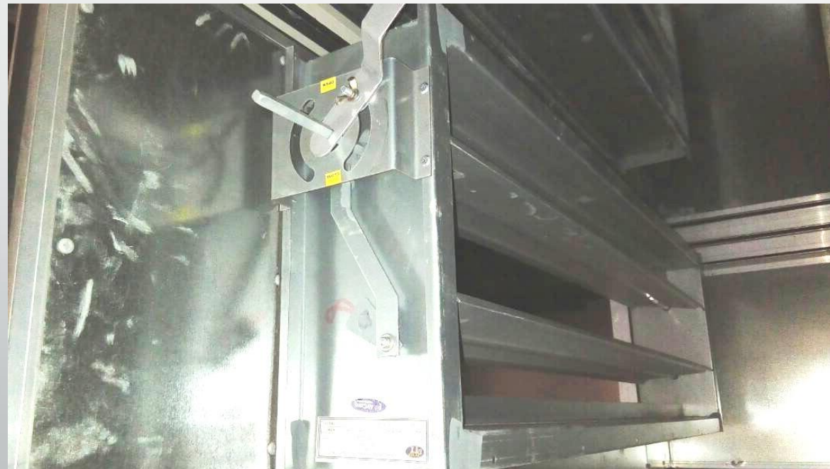
DAMPER INSIDE THE BYPASS BOX
