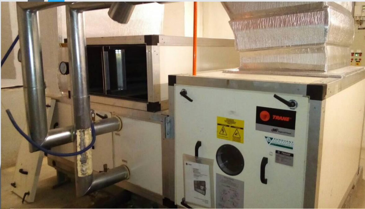
AHU WITH BYPASS DAMPER
